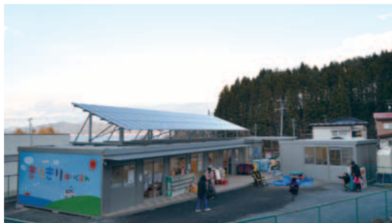
Completed temporary facilities
