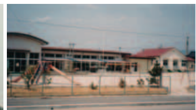
The old Ikkejima Nursery School (Kesenuma Mothers Home was built next to the nursery school)
