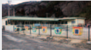
Completed temporary facility © JCU/KO SASAKI
