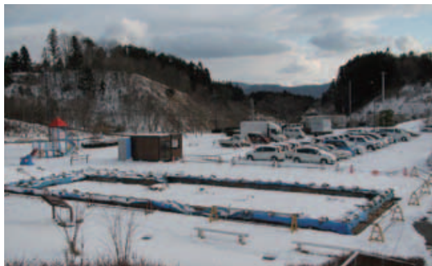
Construction site of the Shizukawa Health Care Center.
